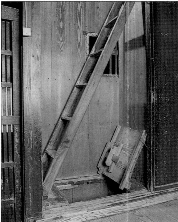
A narrow ladder with trap door beneath in the ninja house at Koga.
