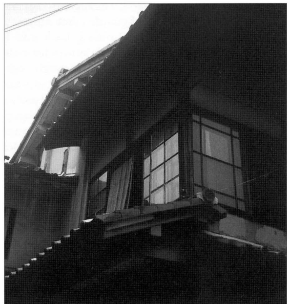
The upstairs window of Nijo jinya in Kyoto. The glazing is a modern addition.
